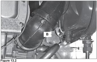
3 Check the pre-load pressure and refer to the section Expansion vessel in the User manual and installation instructions for the correct value.
